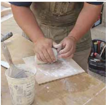
**Prepare the putty.** Knead the putty to an even consistency. Mix in as much additional chalk as necessary to make the putty feel tacky but workable without sticking to your fingers.
