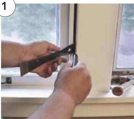
**Dent prevention.** Cut any paint or caulk between the interior stop and window frame with a utility knife. Then, pry the stop free using a putty knife to protect the frame. If there is a nail near the top miter, cut it with an oscillating multitool before trying to pull out the stop.
