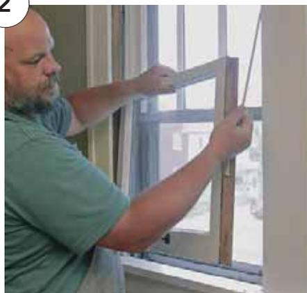
**Remove and inspect the cord.** The sash cord is easy enough to remove, but it's worth inspecting its condition and, if necessary, replacing it with new sash cord (not rope, which will degrade in sunlight).
