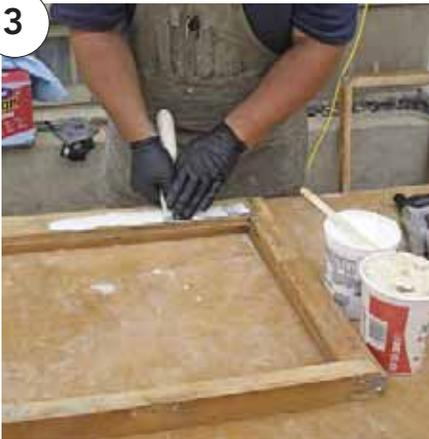
**Fill the damaged areas.** Mix the WoodEpoxy and work it into the repairs with a wide putty knife.
