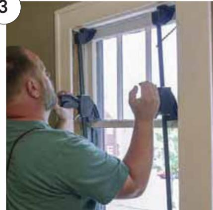
**Upper sashes are often stuck.** Though upper sashes are meant to be mobile, they're often painted shut over the years. Use a pair of bar clamps, reversed to spread apart, to ease the sash free. Place the clamps wide, at the edges of the meeting rail. Otherwise, you may just bend and possibly damage the rail and the pinned bridle joints used to assemble these sashes.
