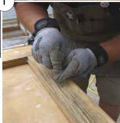
Let the sash dry for about 24 hours after steaming. Then scrape it down to bare wood to get it ready for repairs. In this case, the only issue was minor checking in the wood along the meeting rails. To contain paint chips and dust, set up plastic sheeting on the ground and mist the sash with water to keep dust down while scraping.
