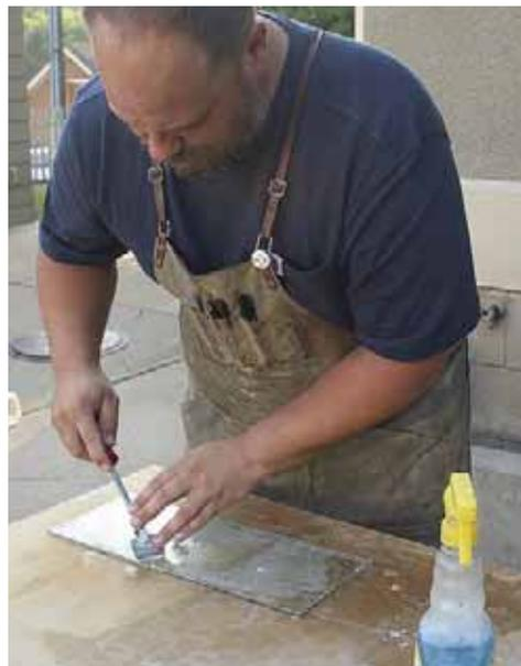
**Free the glass.** Use a putty knife to scrape away the old glazing. Before attempting to remove the glass, make sure all the glazing points are out of the sash. If the putty knife didn't get them out, use a screwdriver or pliers to pry or pull them. Finally, lift the glass from underneath and carefully set it aside.
