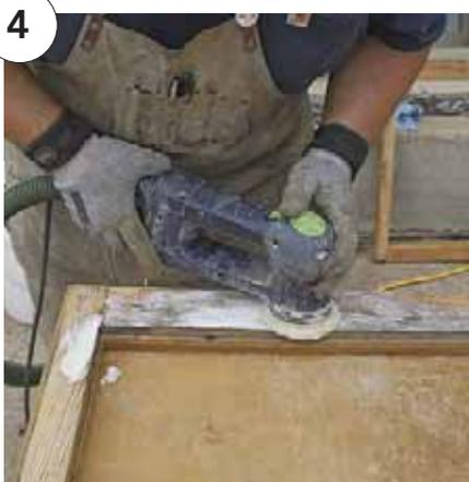
**Sand it smooth.** Allow the epoxy to set for about 24 hours and then sand it smooth with an orbital sander. Run the sander over the entire sash at this point to prepare it for primer.
