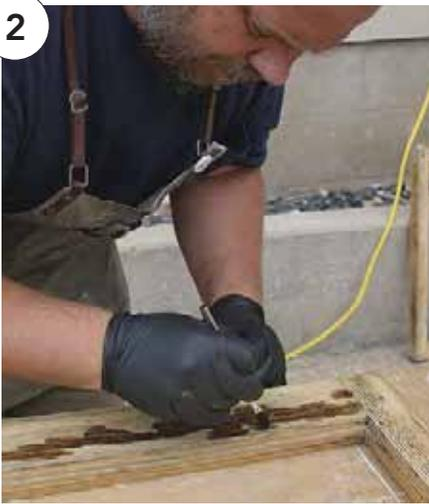
**Penetration, not puddles.** Brush on the LiquidWood epoxy liberally, but only in the area in need of repair. Wait for it to penetrate the wood. The area should look wet, but there should not be puddles.
